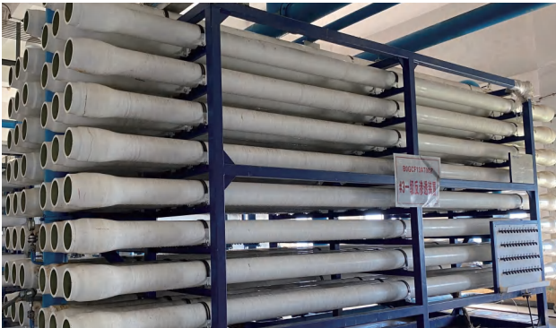
Sea water desalination system of a power plant of Ewindpower Group in China
